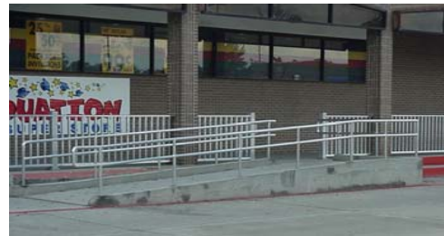
Handrail with handicap access rail
